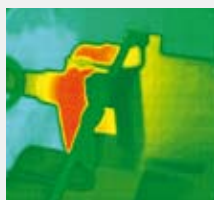
Motor: Bearing Problem
