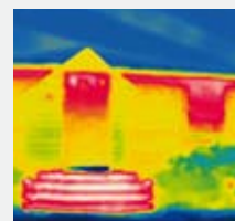
Building: Heat Loss
